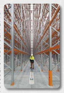
The floor was constructed as a series of large bay post-tensioned floors, coupled together so that there were only two opening joints located within the 25,000  $\mbox{m}^2$  (267,500  $\mbox{ft}^2$ ) ground floor. Combined with the use of a new system for concrete floor jointing—the Rhino joint—this creates a surface that would require little to no maintenance during the life of the structure.
