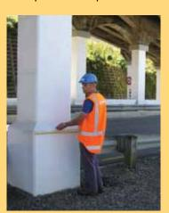
In the three-month project, BBR Contech repaired and strengthened an additional 65 columns, applying one layer of SikaWrap-930G followed by a coating of crack-bridging paint to provide essential protection against the elements. Checks of the FRP jackets installed in 1996 revealed they were still in good shape, providing confidence that this was a high performing and effective long-term total solution.
